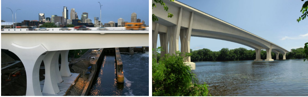
Examples of Broadly Arched Girders and Expressive Piers (MNDOT)
