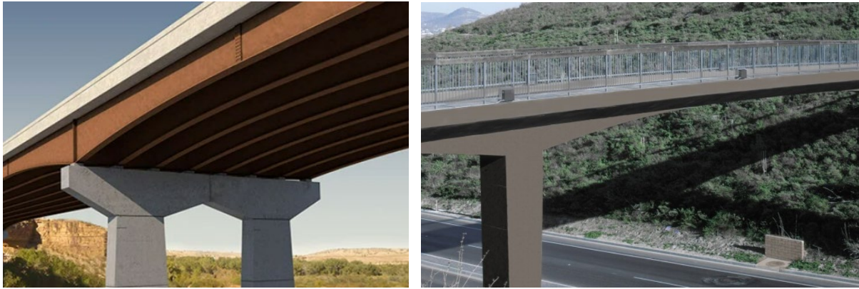
Haunched Weathering Steel Girders and Haunched Integral Color Concrete Girders
