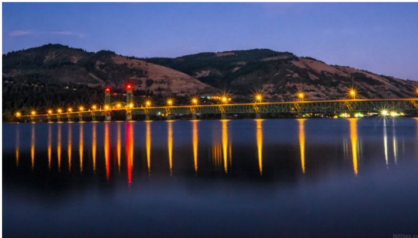
Roadway lighting on the existing bridge
