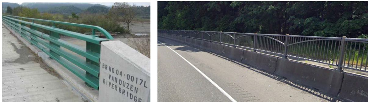
Example of a steel traffic barrier (CALTRANS) and the Historic Columbia River Hwy. barrier
