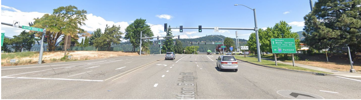
Button Bridge Road, Hood River Existing Condition
