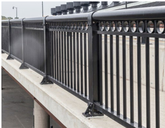
Examples of traditional and industrial style, highly transparent and climb-resistant railings.
