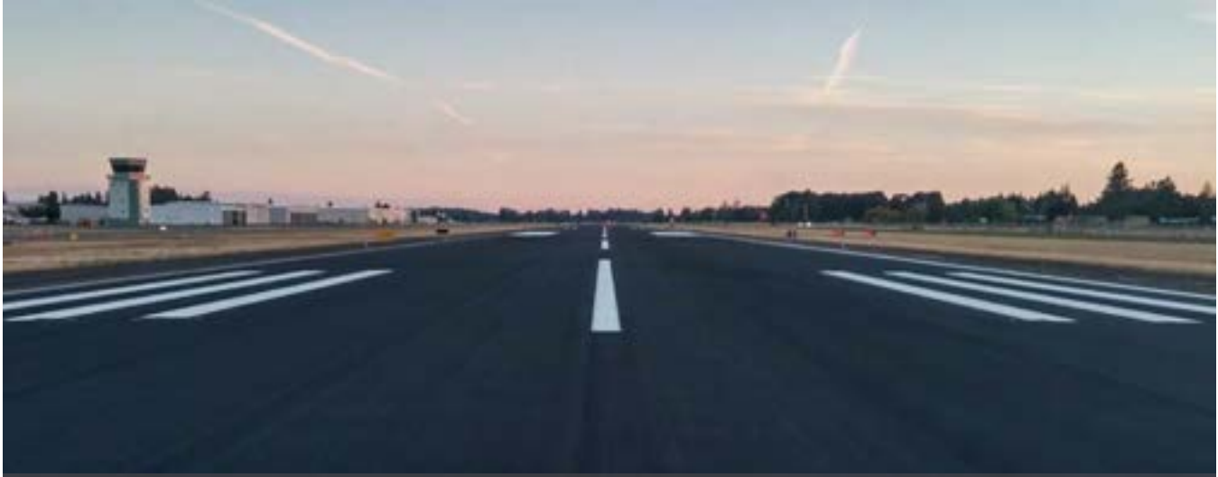
Runway 17 Looking South – Source: Century West Engineering
