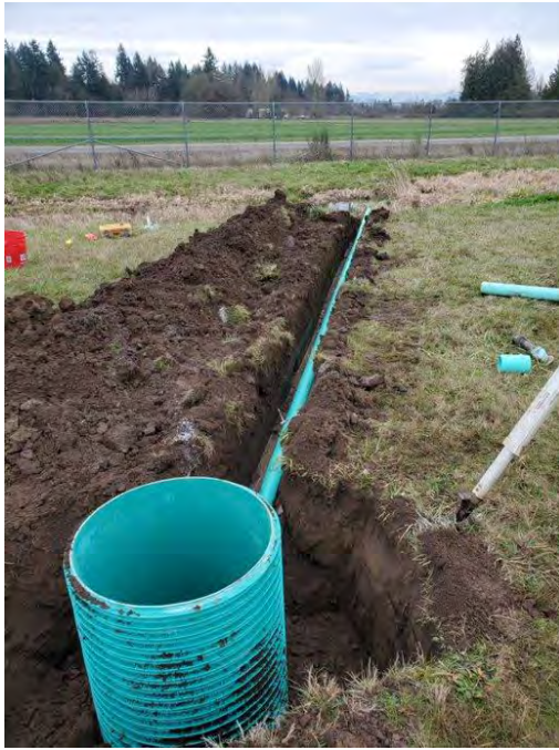
Figure 4 –24" silt traps were installed at the inlet end of each tight line outfall, which discharged toward existing drainage swales on the site. Photo taken facing west toward the west property line (fence) with Hubbard Cutoff Rd. NE in the background.
