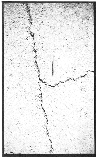
ASPHALT CONCRETE RUNWAY PAVEMENT SHOWING TYPICAL LONGITUDINAL AND TRANSVERSE CRACKING (NOTE 6-INCH PEN NEAR CRACK INTERSECTION)
