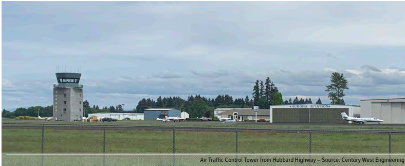
Air Traffic Control Tower from Hubbard Highway – Source: Century West Engineering
