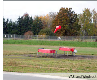
Source: Century West Engineering
