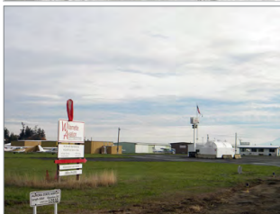
Willamette Aviation Fuel Tanks
