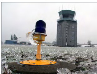
Taxiway Light and Air Traffic Control Tower
