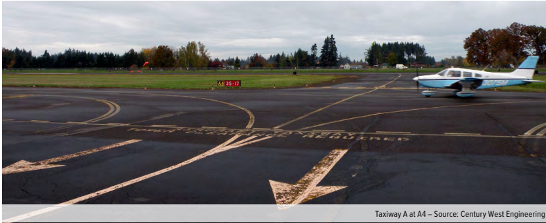
Taxiway A at A4 – Source: Century West Engineering
