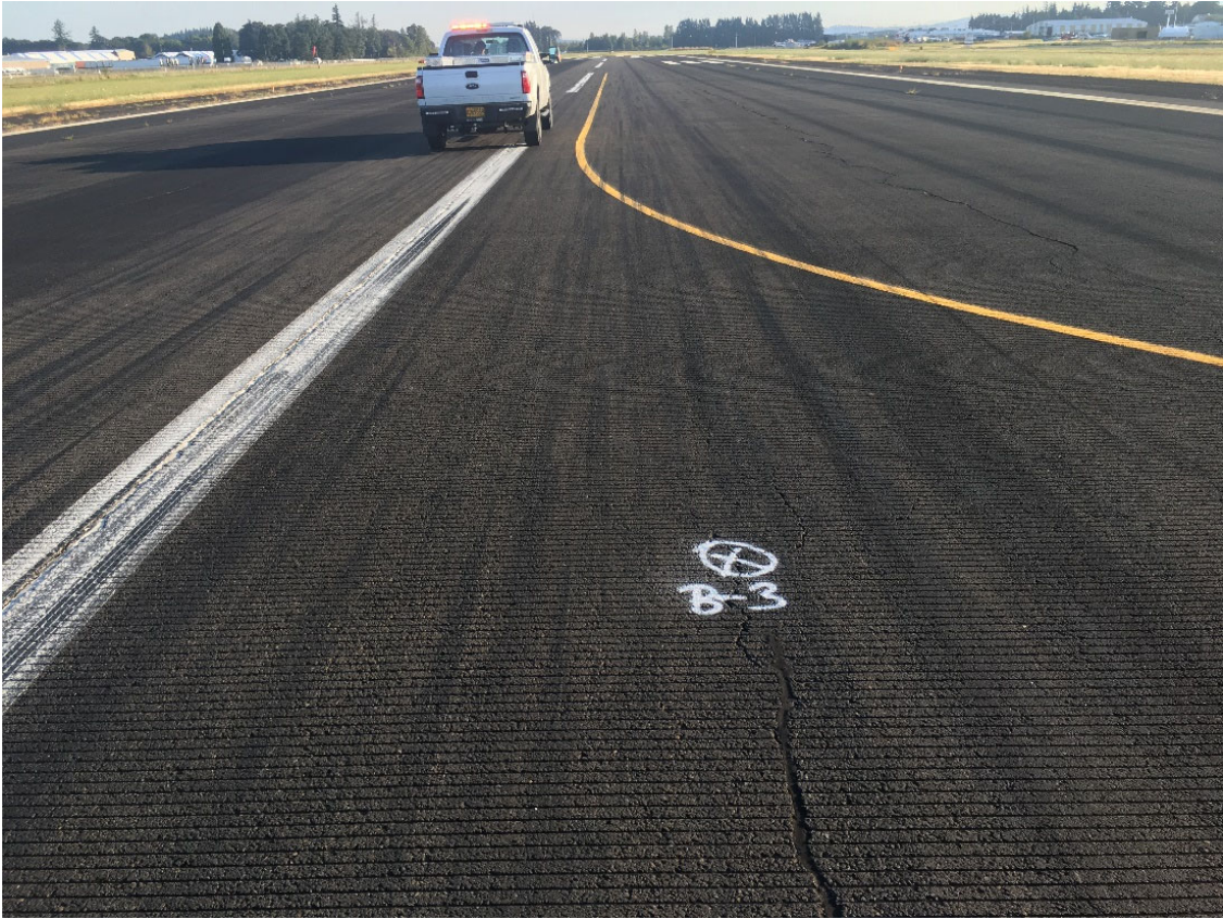
Core B-3 (RW 17-35 12' East of Centerline, Station 19+41, FWD 32)
