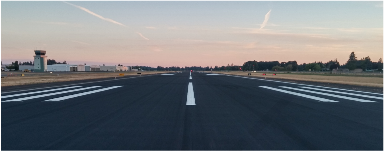
Runway 17 Looking South – Source: Century West Engineering
