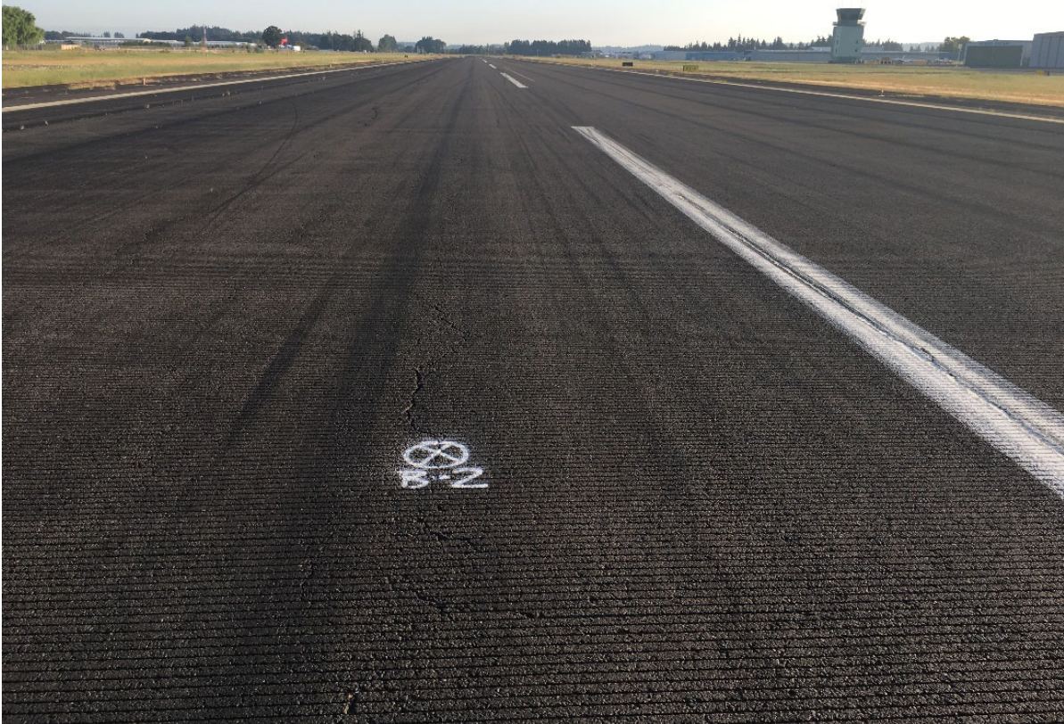
Core B-2 (RW 17-35 8' West of Centerline, Station 39+51, FWD 16)
