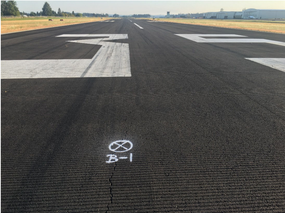
Core B-1 (RW 17-35 8' West of Centerline, Station 56+81, FWD 26)
